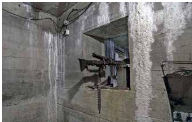
Machine gun (contemporary but not original) within one of the guardrooms which protected each entrance at Rzeczka. Photo Chris Wilkins
